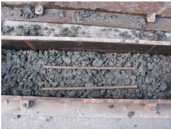
Fig 2: 2-8 mm Ø Bar placed at center from all direction of beam
