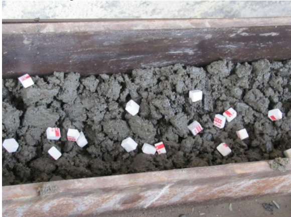
Fig 1: Rubber anomalies mixed with concrete
